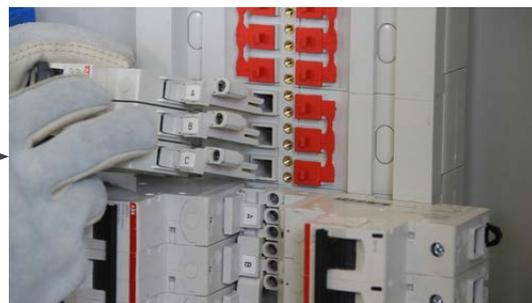
The Breaker Is Inserted Into The Opening
